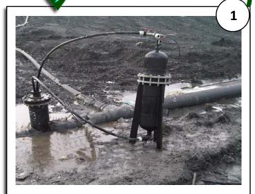
The **Silt Pro** II was set up on site quickly with minimal fuss and began the process of removing silt from the Knock Out Pot whilst the system remained live! This represents a considerable cost saving as no gas engines had to be turned off - unlike alternative methods of de-silting!
