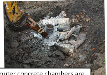
The outer concrete chambers are then broken up and the in-situ formed concrete infill also broken down.
