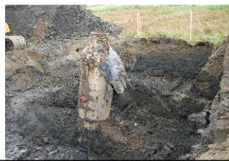
After careful excavation the concrete rings are exposed to allow the overall well height to be reduced.
